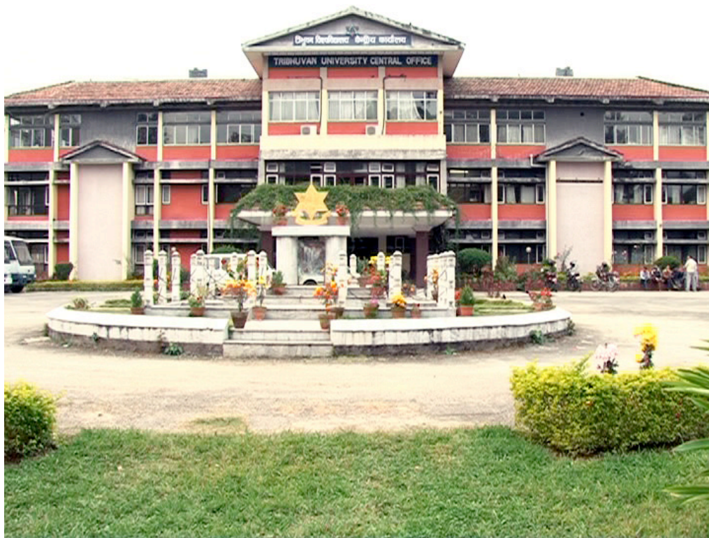
Fig. 52 The Tribhuvan University Administrative Building ((NET-56).
