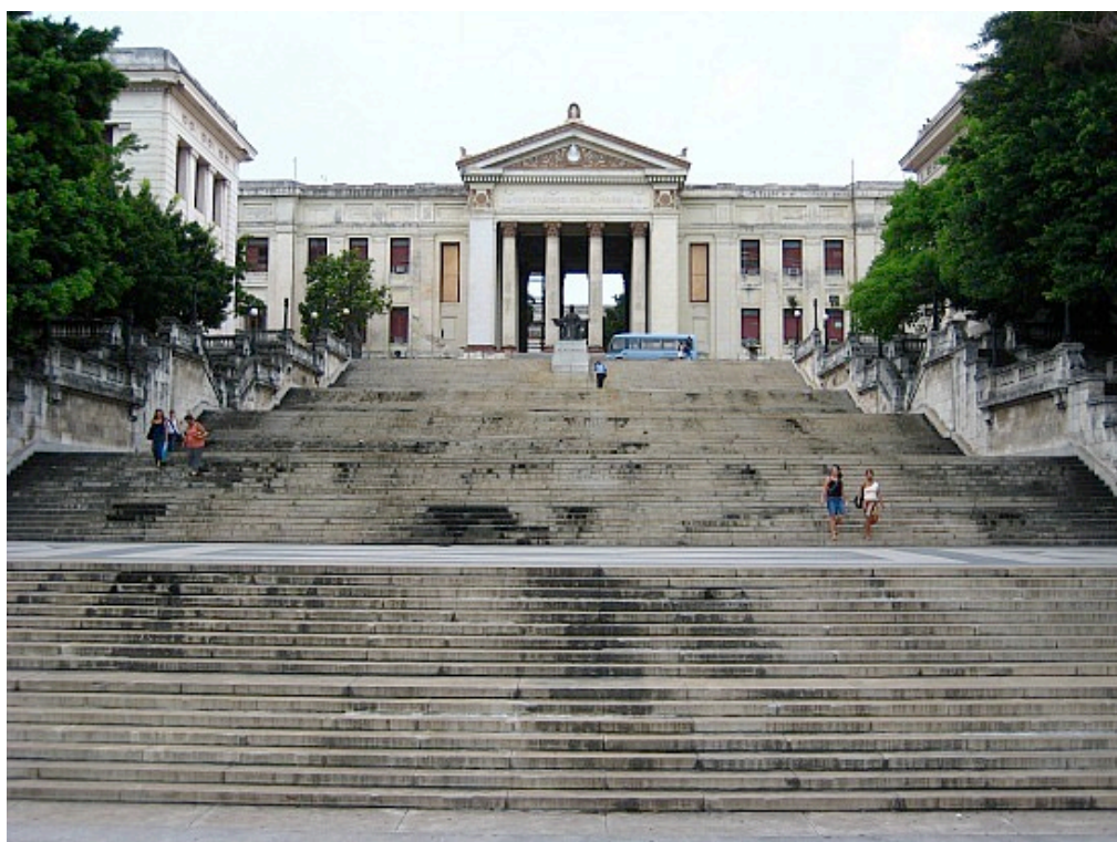
Fig. 57 The University of La Havana, where the Latin American Network of Ferroelectric Materials has its main node (NET-43). Credit: Ismael Clark Arxer, UNESCO Science Report 2010
